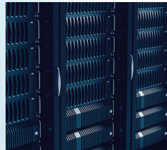
Cloud Data Center
